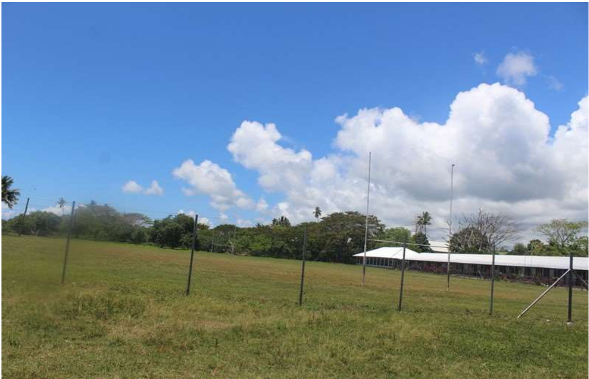
Fasito'otai Secondary School and rugby field located within Coastal Hazard Zone
