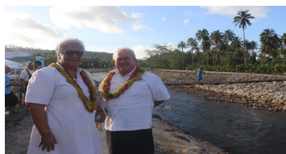
The River Protection Rock Wall at Lalomauga. Deputy Prime Minister, Fiame Naomi Mataafa carried out the ribbon cutting of the ceremony.
