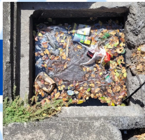
MOTO'OTUA DRAINAGE SYSTEM UP ROAD
