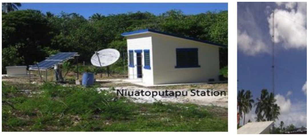
Figure 6 Existing Seismic Station infrastructure in Niuatoputapu and Tongatapu, Tonga
