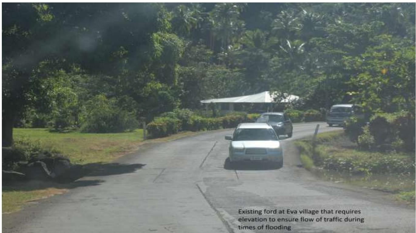
Existing ford at Eva village that requires elevation to ensure flow of traffic during times of flooding
