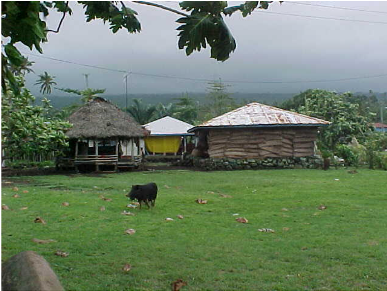
Buildings in CFHZ at Vailoa showing raised floor levels to avoid flood hazard.
