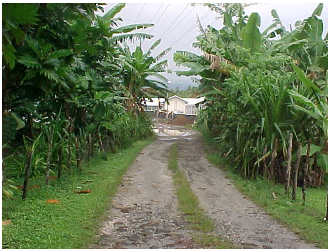
Access road to new church and school unformed and subject to flooding.
