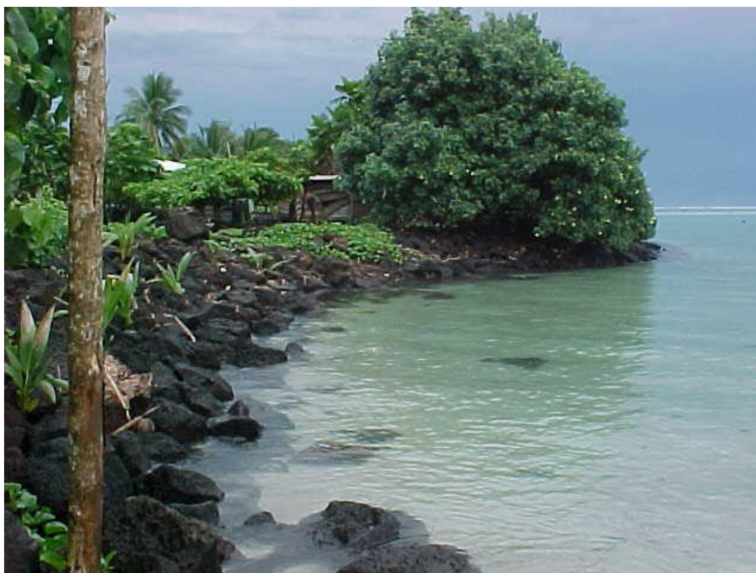
Seawall at Sale'aula in good condition follows original coastline. Area behind seawall built up for new Main Road with dredgings from the lagoon.
