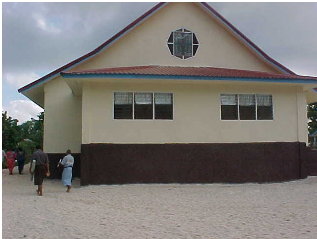
The back of the church is built up about 2 metres above the surrounding ground level to avoid the flood hazard.
