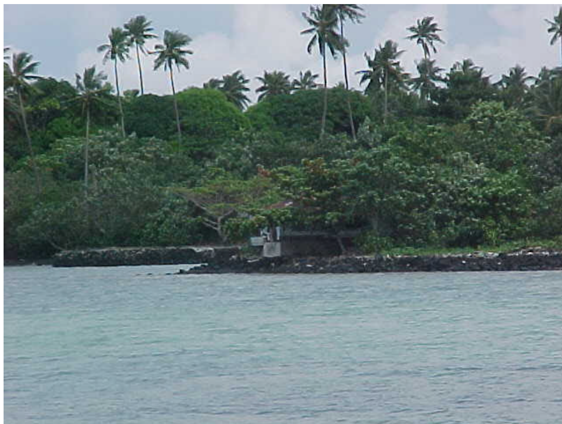
Coastline at Satalafai looking south. Typical rocky headlands with minor reclamations or builtup areas and small rock protection.
