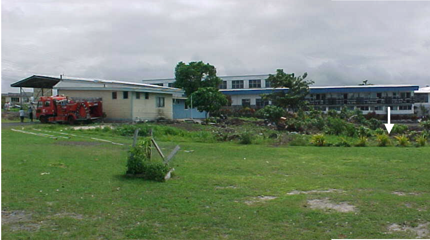
Fire Engine and Transport Control Board offices located in Coastal Erosion and Flood Hazard Zones. Approximate edge of inlet from the lagoon shown arrowed.
