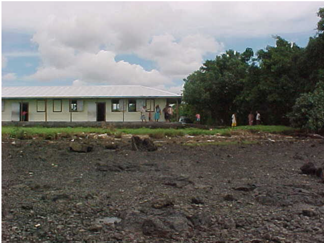
Front of Primary School approximately 10m from beachfront.
