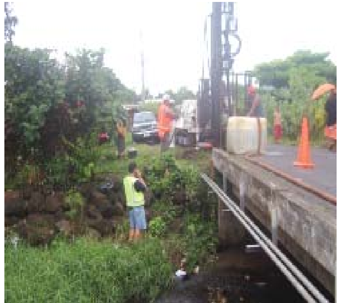
Men at work....drilling
