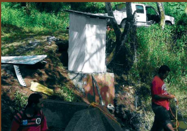
The completed flow gauge housing
