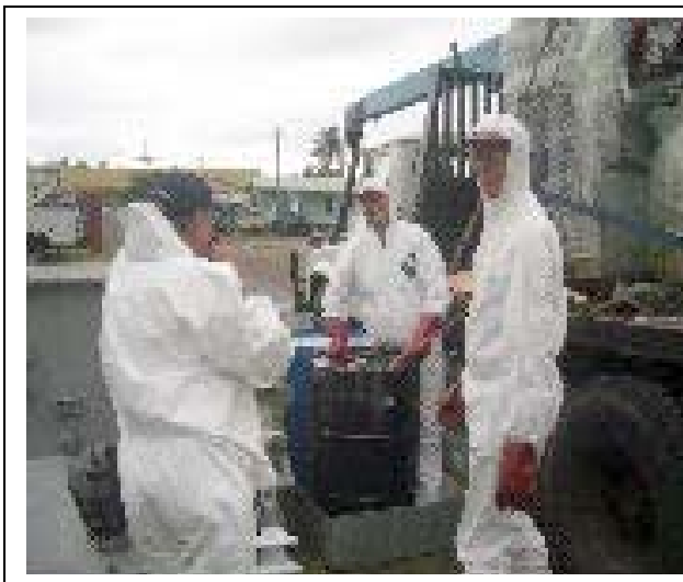
Figure 3: Two AMC consultants and Project Coordinator POPs draining PCB-contaminated transformer oil from Savaii. Photo: MNRE.
