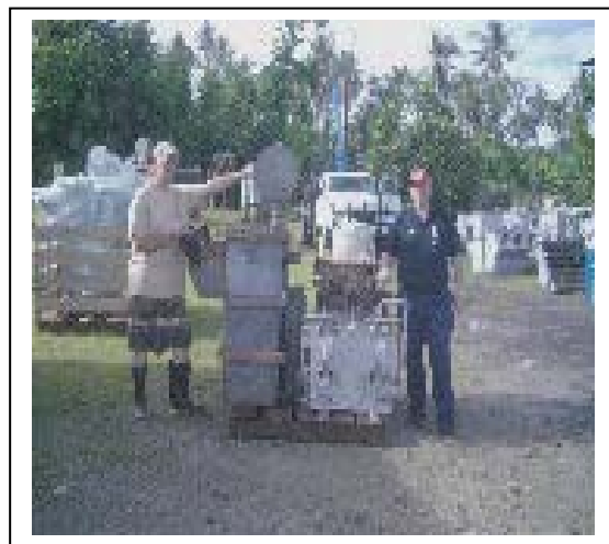
Figure 8. Drained Contaminated Transformers on pallets prepared for disposal. Photo: MNRE
